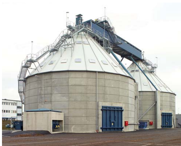
SRF storage silos are available in sizes up to 5,000 m 3
